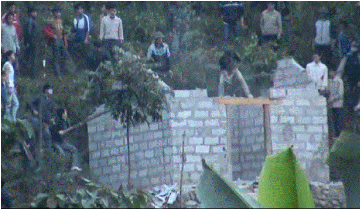
Picture 21: Demolition of the funeral storage shed in Hamlet Khuoi Vin on Nov 24, 2013
